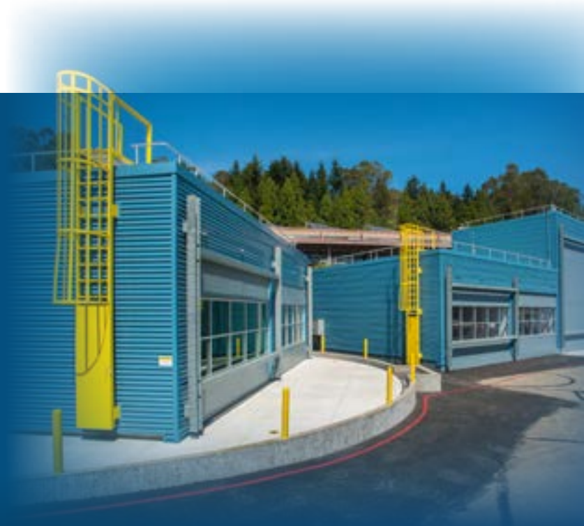
FLEXLAB test bed XR, on its rotating turntable, is on the left.
