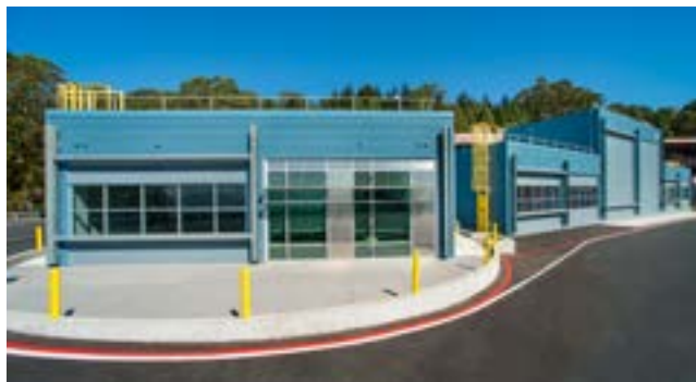
FLEXLAB is located at Lawrence Berkeley National Lab
